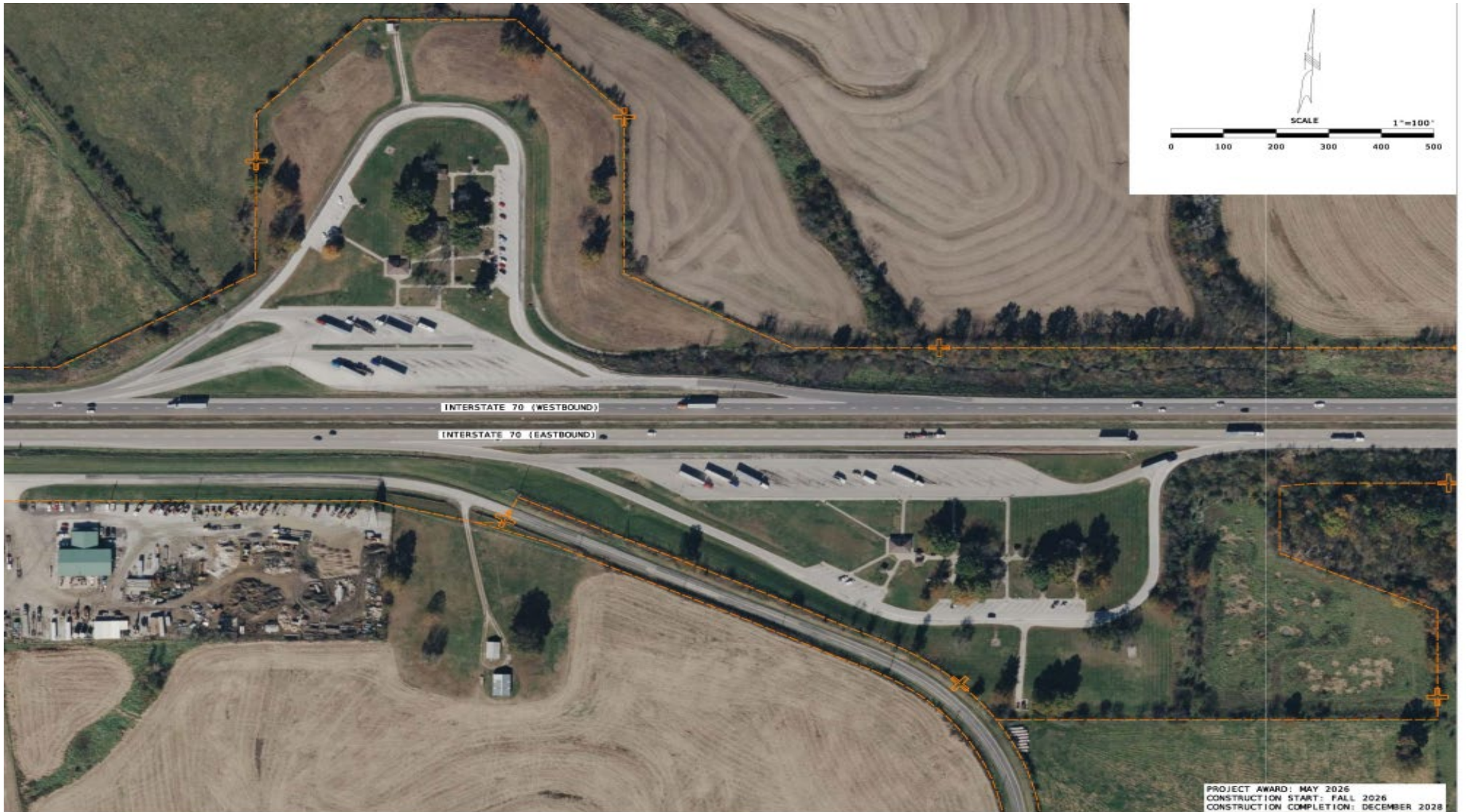
BOONVILLE EASTBOUND & WESTBOUND (MM 104)
